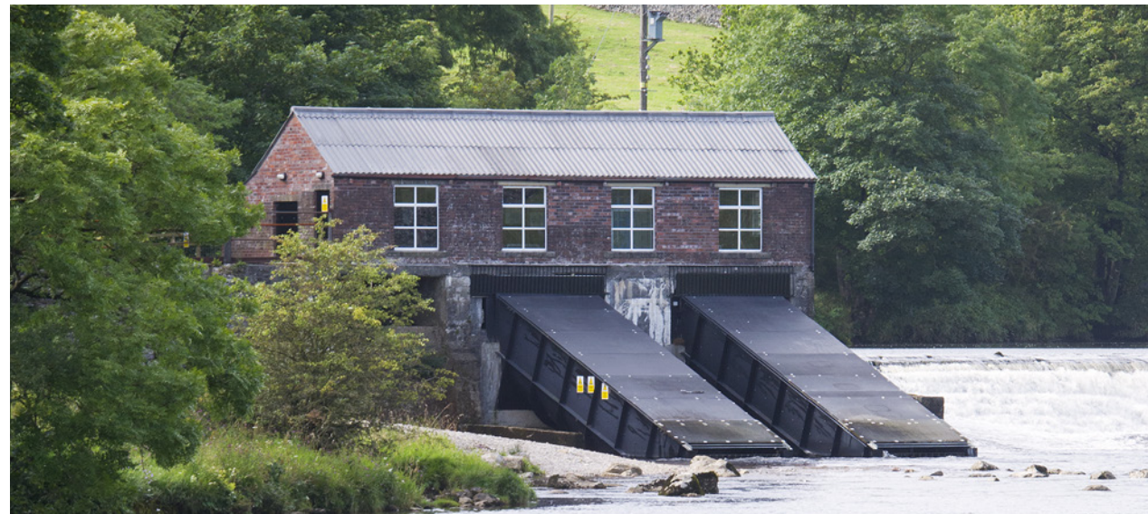
Renewable energy: Linton Falls is a scheduled monument that has found an economic future by reverting to its original use as a hydro-electric power station
